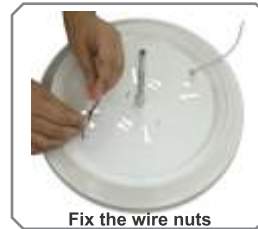
Fix the wire nuts
